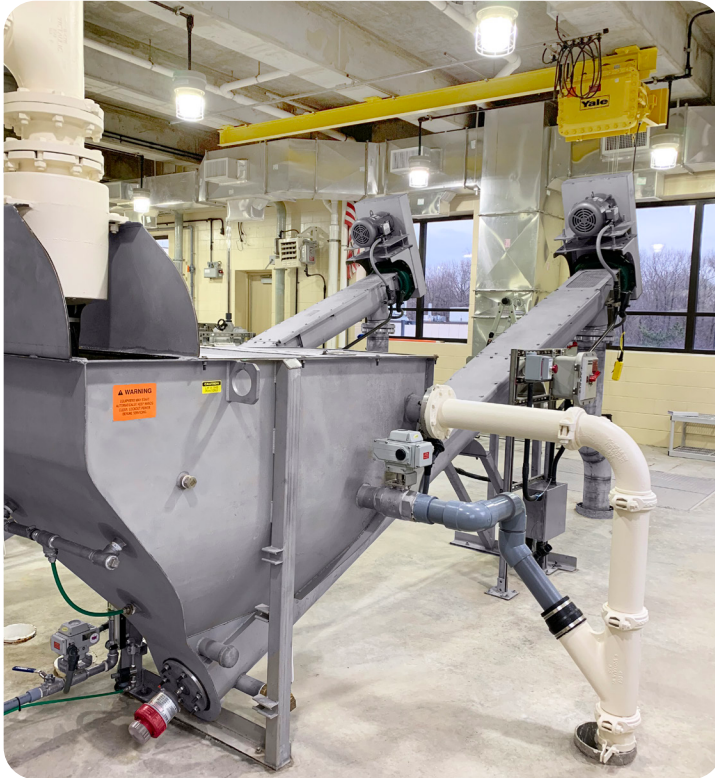
Sleek in design, the PISTA® TURBO™ Grit Washer with TRI-CLEANSE Technology™ works in concert with the PISTA® Grit Concentrator to produce clean, dry grit.
