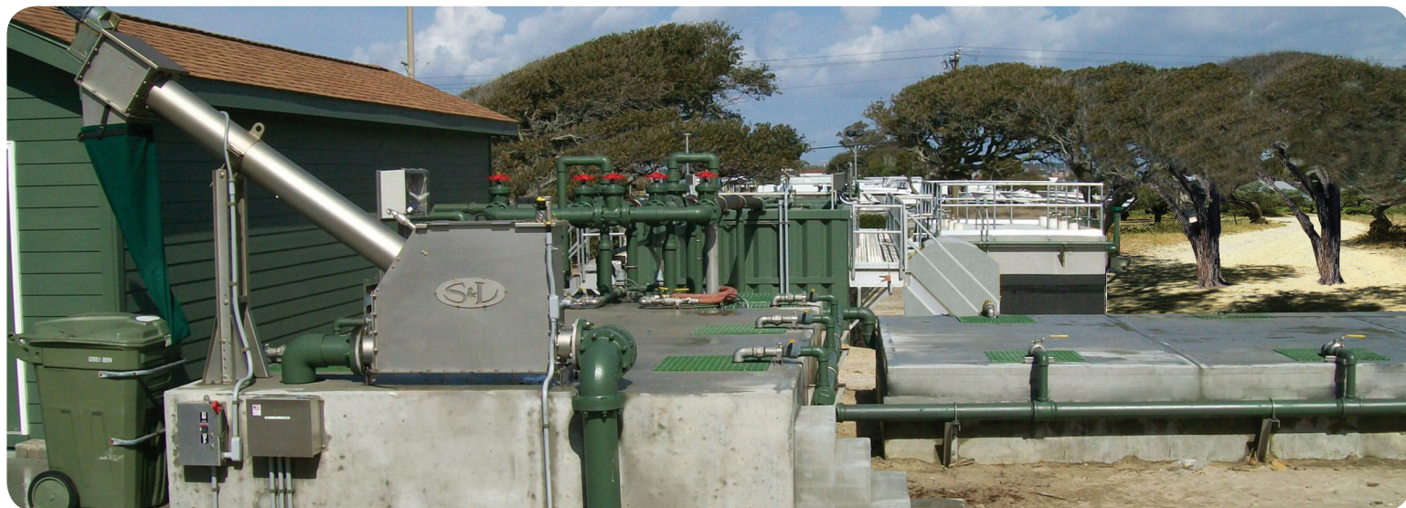
Waste from residents of a condominium complex in North Carolina is separated by the OBEX™ Spiral Fine Screen (at left of photo), then sent on to the TITAN MBR™ for treatment (in the background) .
