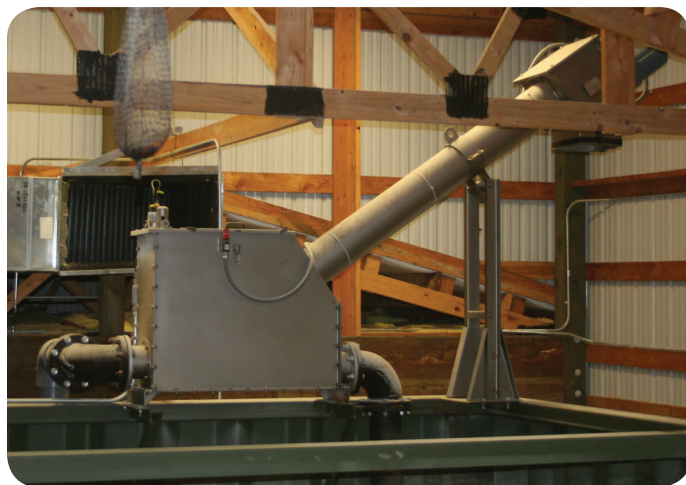
The OBEX™ Spiral Fine Screen can be mounted on any flat surface, including the side of this TITAN MBR™ treatment system.
